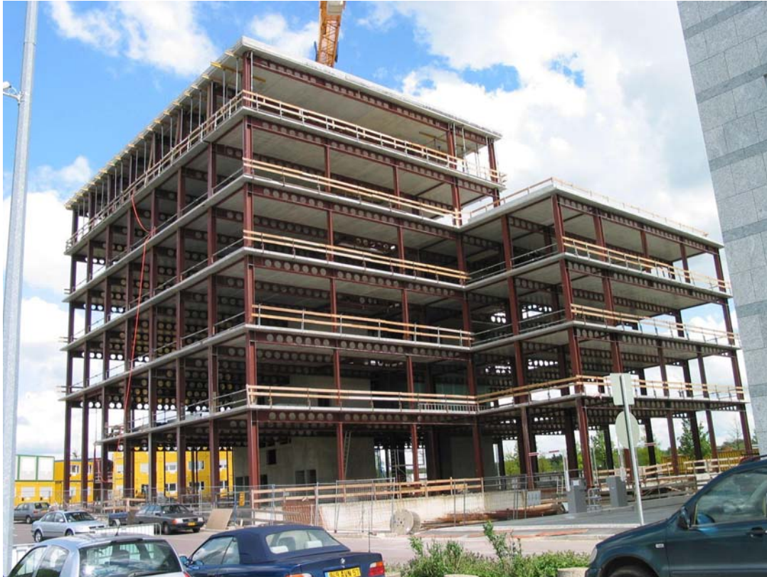
Figure 42. "Banque Populaire" with steel frame and concrete floors completely erected in June 2002.
