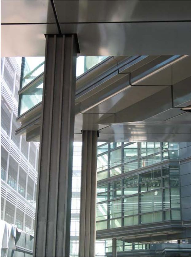
Figure 48. "Chambre de Commerce" with visible, unprotected steel columns on ground level.
