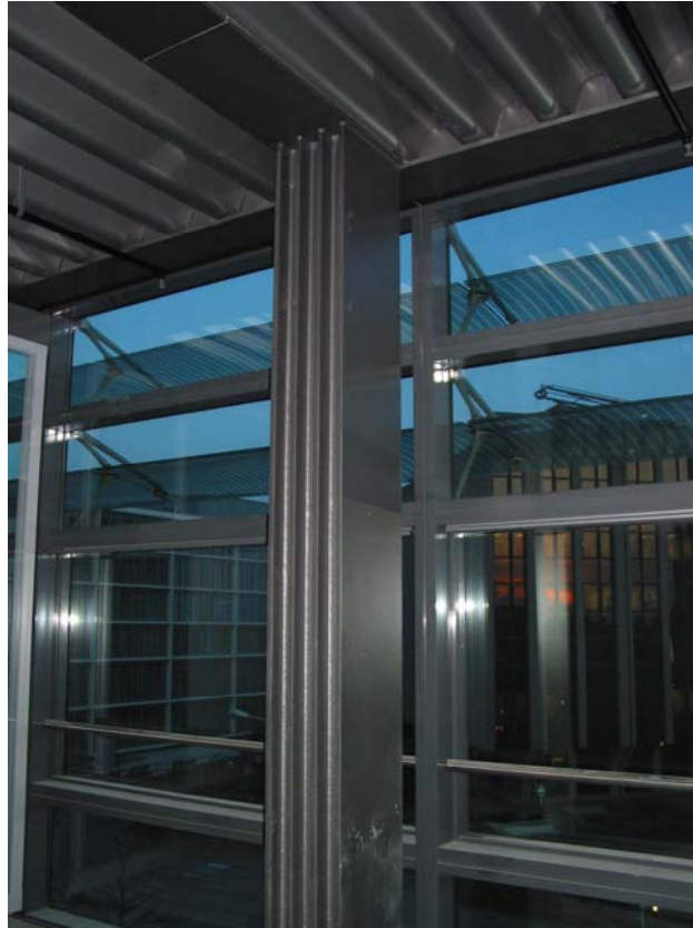
Figure 46. "Chambre de Commerce" with visible, unprotected steel columns supporting the composite beams.
