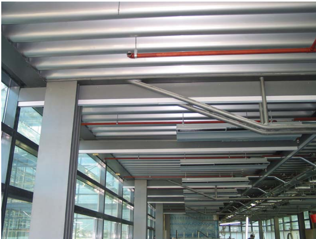
Figure 47. "Chambre de Commerce" with composite beams sustained by visible, unprotected massive tension rods.
