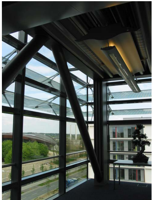
Figure 49. Building C with lateral steel bracing.
