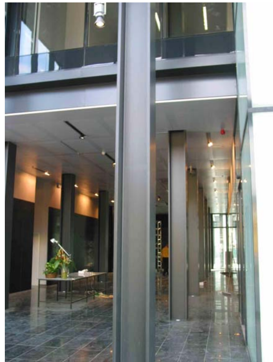
Figure 44. "Banque Populaire" with entrance hall and visible, unprotected steel columns in July 2003.
